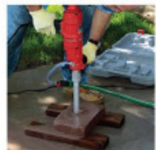
add pressure and drill through paver.
