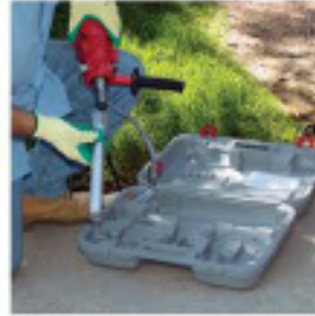
Attach Diamond Core Bit
