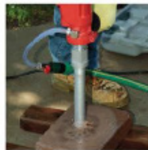
As drill bit gets started, straighten to 90°
